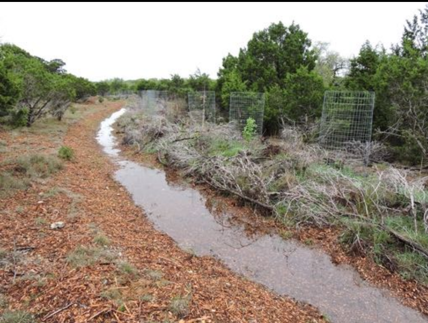
NEW HILLSIDE CONTOUR BIOSWALE
